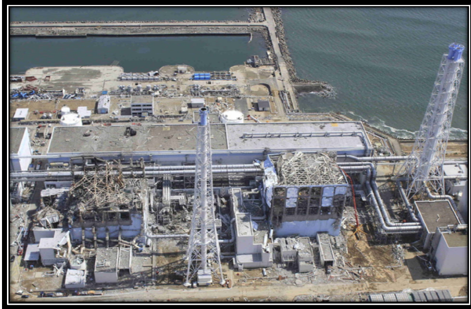
Figure 3 Damaged reactor buildings of Units 3 and 4 caused by hydrogen explosions on 14–15 March (NAIIC, 2012) (photo: Air Photo Services, Japan)
