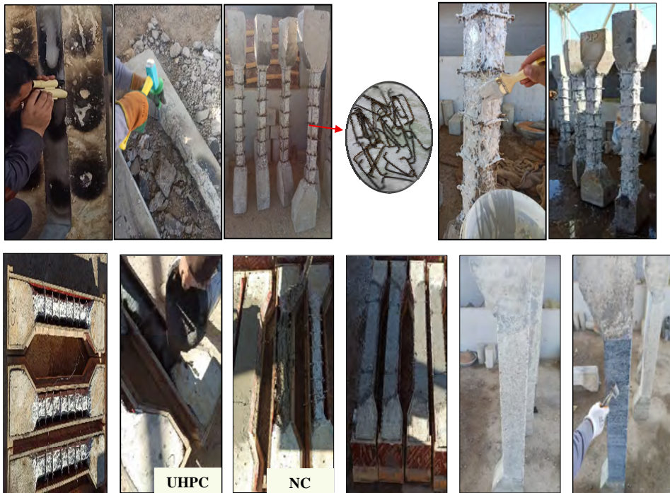
Figure 8 Sequential steps of RC column repair (see online version for colours)
