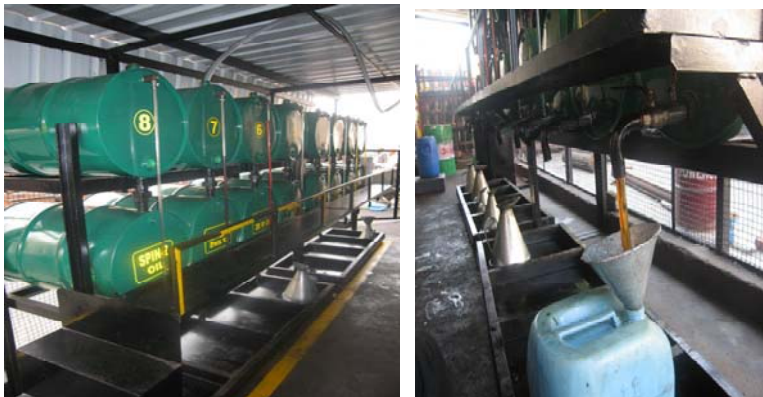
Figure 11 Storage drums of different oils and new pouring systems of oils (see online version for colours)
