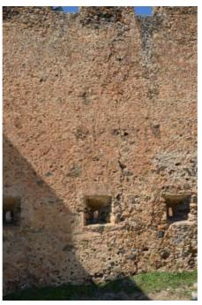
Figure 6 Vertical, through and through crack in the east wall: internal view (see online version for colours)
