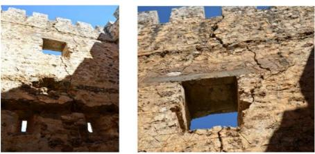
Figure 5 Vertical, through and through crack in the east wall: external view (see online version for colours)
