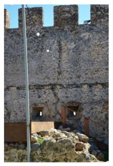
Figure 7 Crack in the north face, north east tower (see online version for colours)
