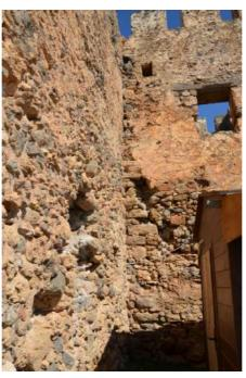
We can observe similar behaviour to the southeast tower, with cracks on the east side (Figure 9) and disruption of the masonry at lower levels. The cracks in this specific region are due to the out of plane bending of the masonry and shear failure, which begins from the opening and appears at the region, where we have reduction of the cross-section (see, architectural plans, where the south wall's thickness is 1.4 m and the east and north wall's is 0.77 m).
