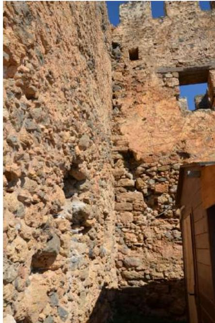
We can observe similar behaviour to the southeast tower, with cracks on the east side (Figure 9) and disruption of the masonry at lower levels. The cracks in this specific region are due to the out of plane bending of the masonry and shear failure, which begins from the opening and appears at the region, where we have reduction of the cross-section (see, architectural plans, where the south wall's thickness is 1.4 m and the east and north wall's is 0.77 m).
