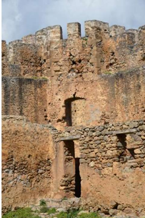
On the north side of the north east tower (Figure 7), another crack appears (partially refurbished), where we can observe the phenomenon of the disruption of the masonry (Figures 8).
