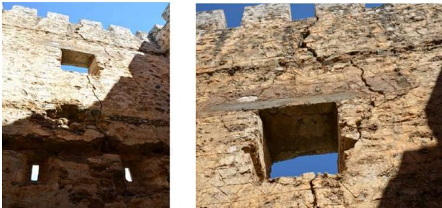
**Figure 5** Vertical, through and through crack in the east wall: external view (see online version for colours)
