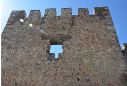
**Figure 8** Disruption of the masonry in the south side, north east tower (see online version for colours)
