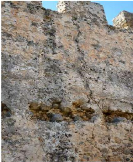
**Figure 11** Disruption of the masonry, in the connection area between the south wall and the south west tower (see online version for colours)
